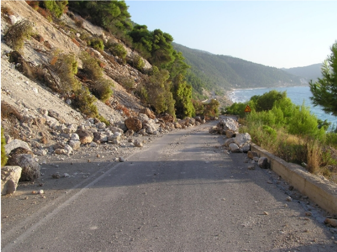
Figure 4. Landslide in Pefkoulia (see location in Fig. 3).
